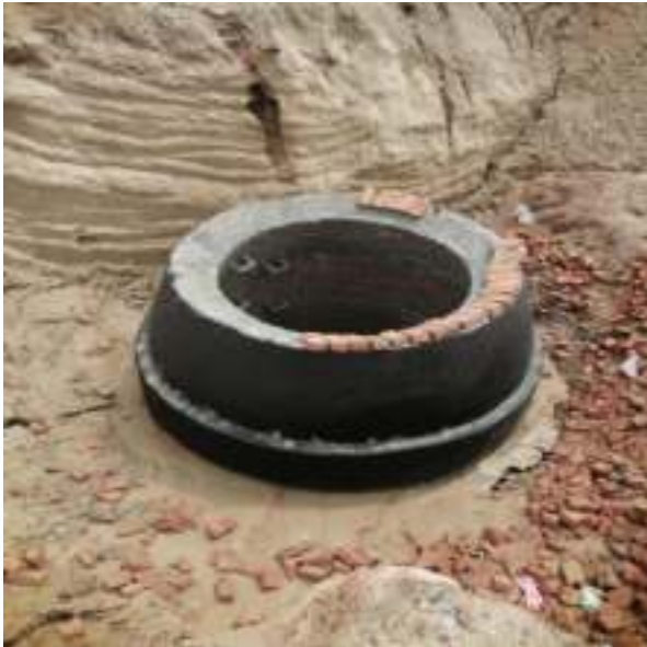
Picture 31: Manhole under Construction
