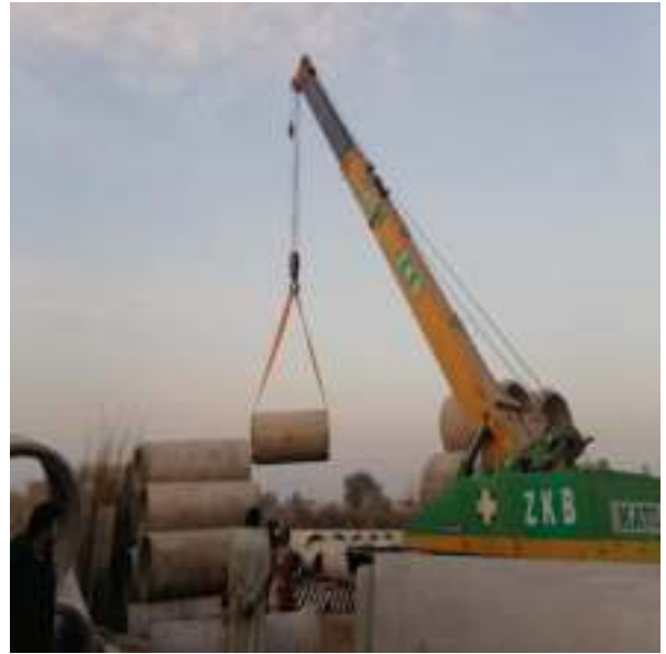
Picture 64: Hauling of Pipe in Progress
