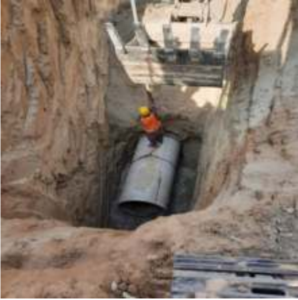
Picture 37: Laying of Sewer Pipe at Harrapa Road
