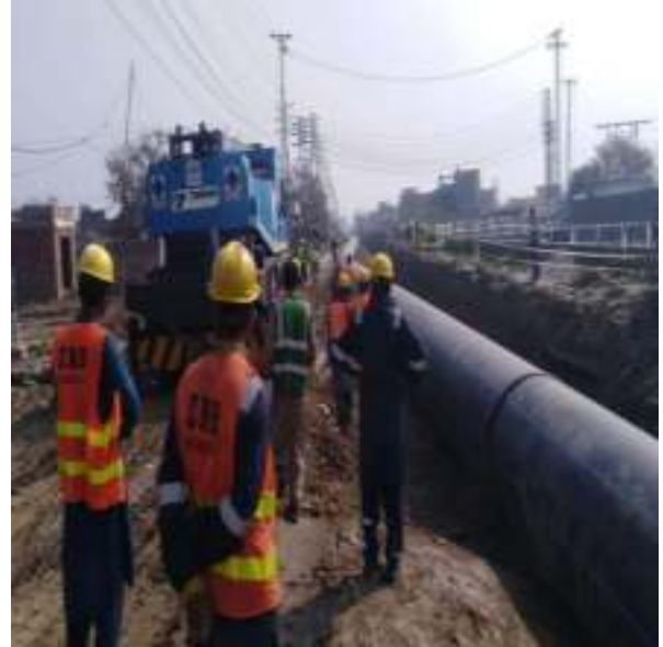
Picture 87: Backfill Restoration
