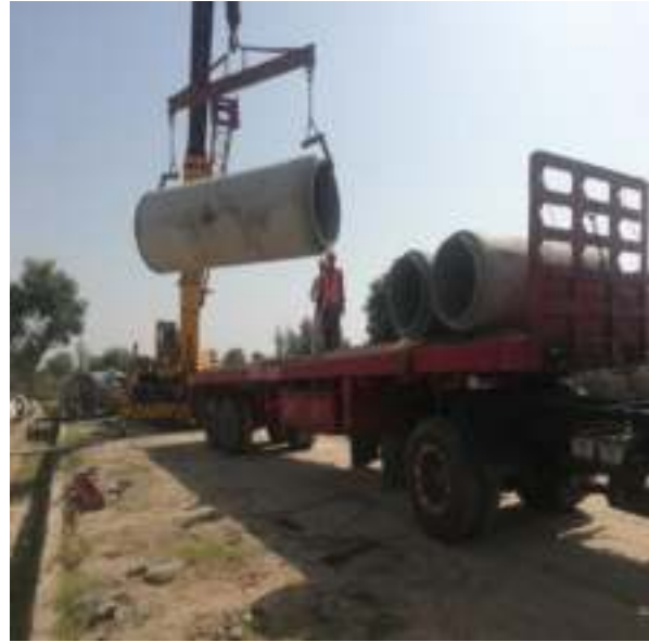
Picture 30: HAULAGE OF RCC PIPES
