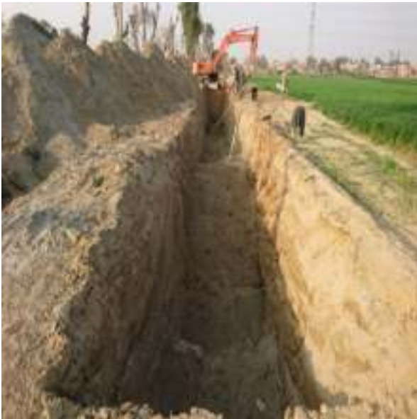
Picture 23: Excavation for sewer laying is in progress
