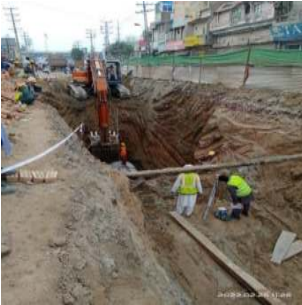
Picture 65: Pipe Laying & Level Inspection in Trench
