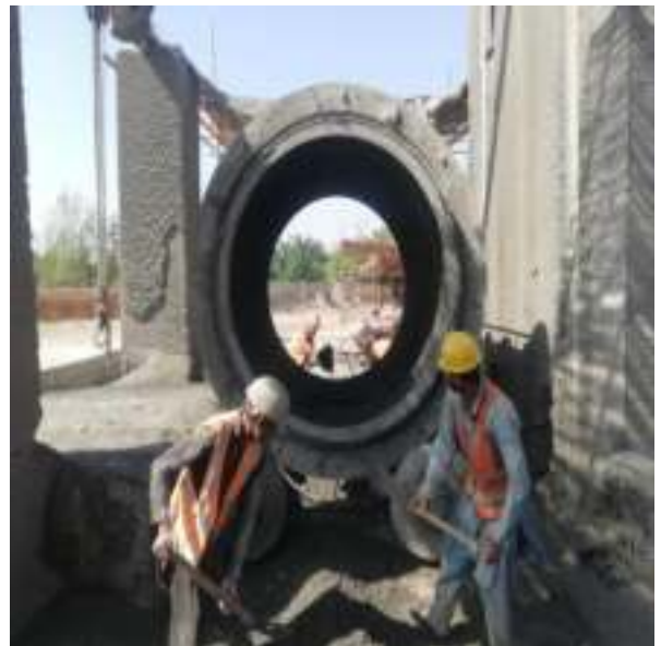
Picture 24: Manufacturing of RCC Pipe
