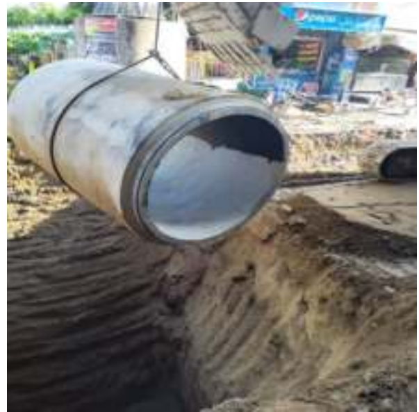
Picture 75: Pipe Laying in Progress
