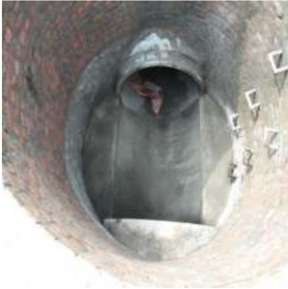
Picture 45: View of Manhole Bed and Manhole Grating
