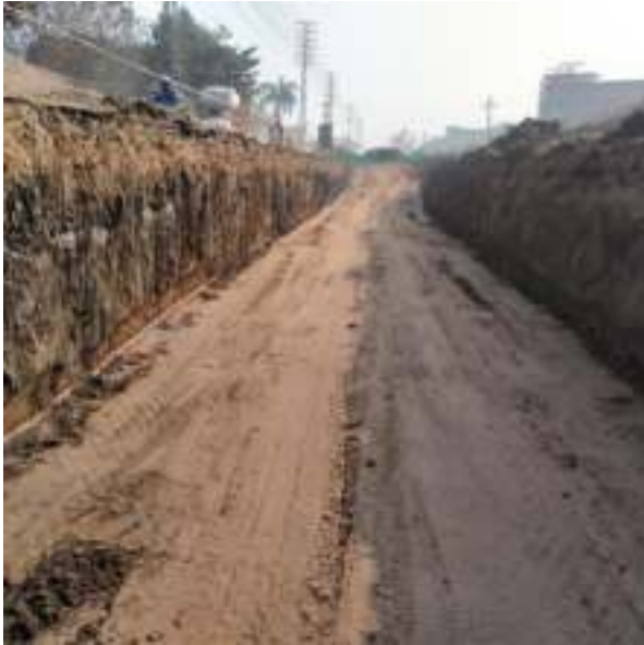
Picture 90: Sewer Bed Preparation
