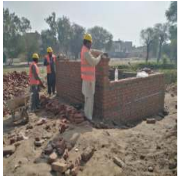
Picture 20: Brick Work at Pump House in progress
