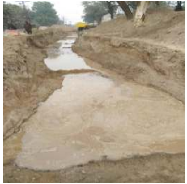
Picture 38: Flooding of Sewer Bed is in progress, Sahiwal Lot-2
