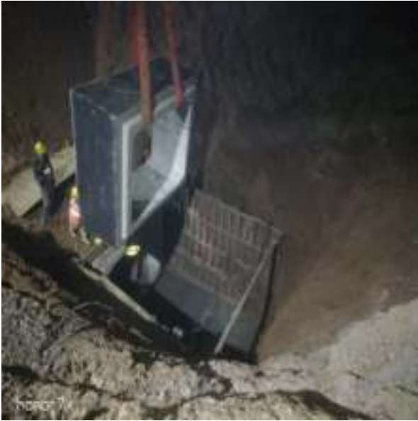
Picture 82: Conduit Placement (Night Shift)
