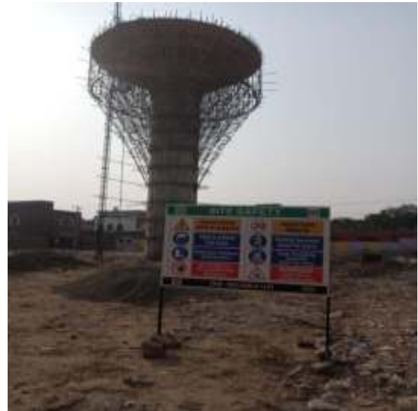
Picture 97: Construction of OHR in Progress
