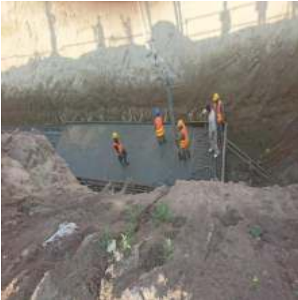
Picture 43: Concrete Roof Slab in Progress, Sahiwal
