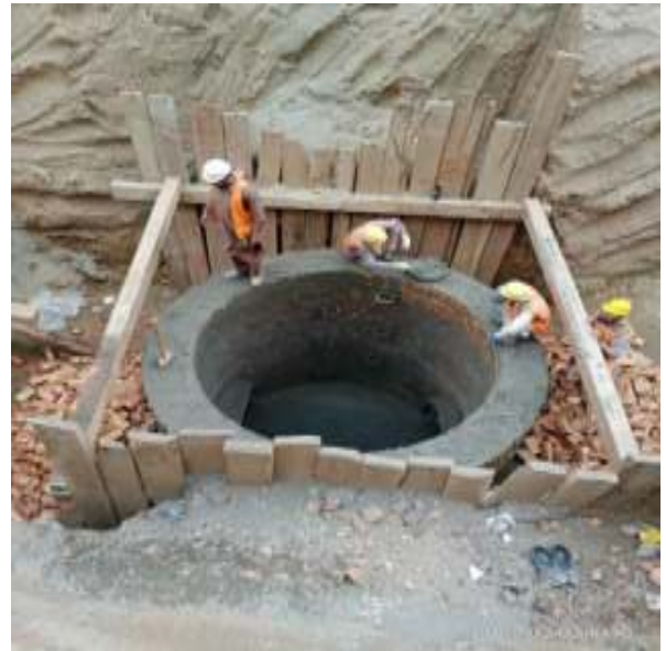
Picture 70: Manhole Construction
