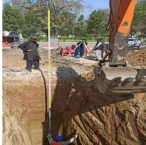
Picture 28: Manhole under Construction
