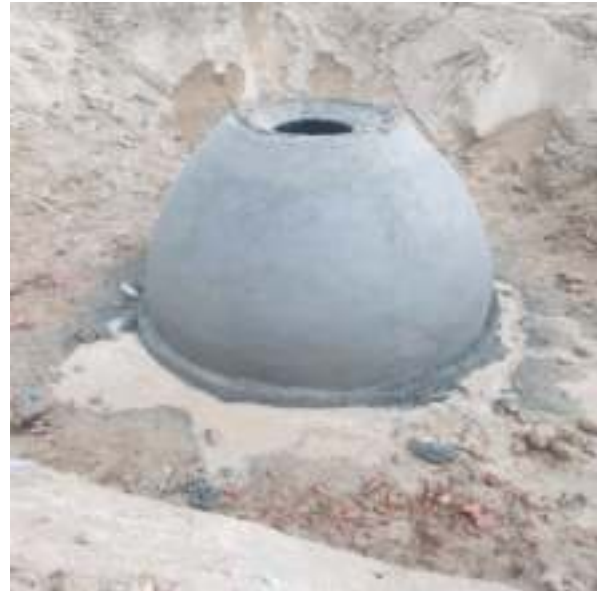
Picture 32: Manhole under Construction
