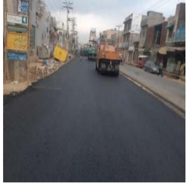
Picture 68: Compaction of Asphalt Concrete Base Course
