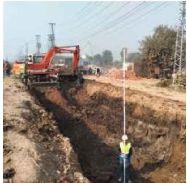
Picture 89: Bed Preparation for layinf of Forcemain
