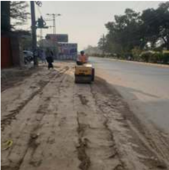
Picture 19: Restoration Work is in Progress
