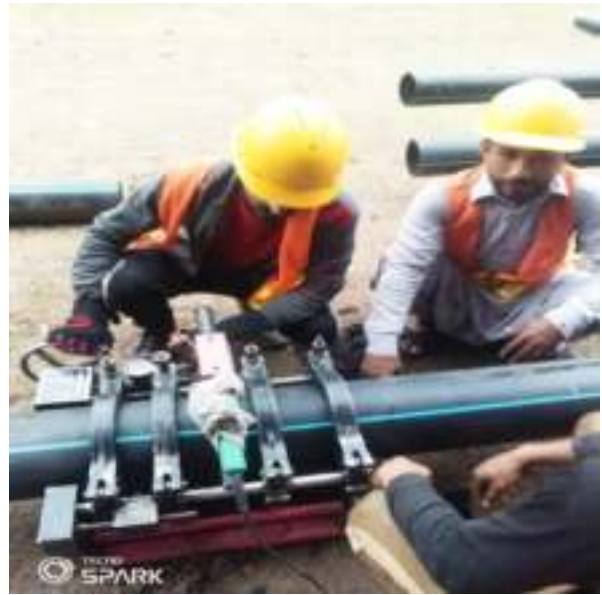
Picture 18: HDPE Pipe Jointing At UC-10
