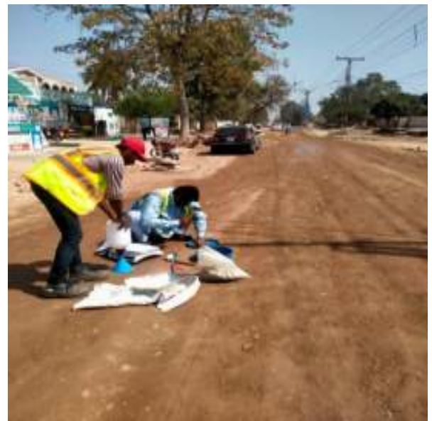
Picture 60: Field Density Test at Road-01
