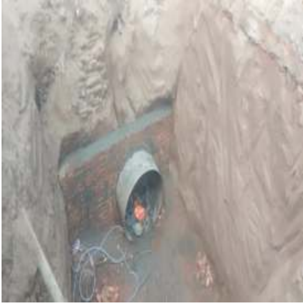
Picture 67: Pipe Laid and backfilled
