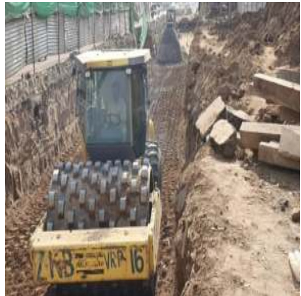
Picture 66: Compaction of Backfill
