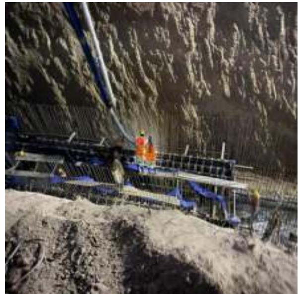
Picture 40: Pouring of Conduit Wall Concrete in Progress, Sahiwal Lot-2
