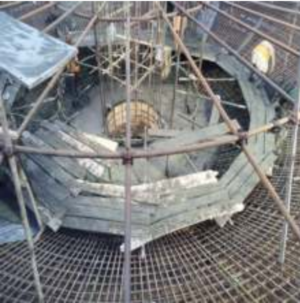
Picture 96: Construction of OHR in Progress
