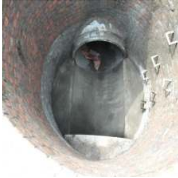
Picture 36: Manhole Benching completed Lot-02
