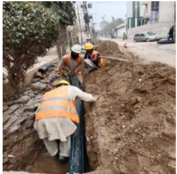
Picture 16: HDPE Pipe laying in Progress
