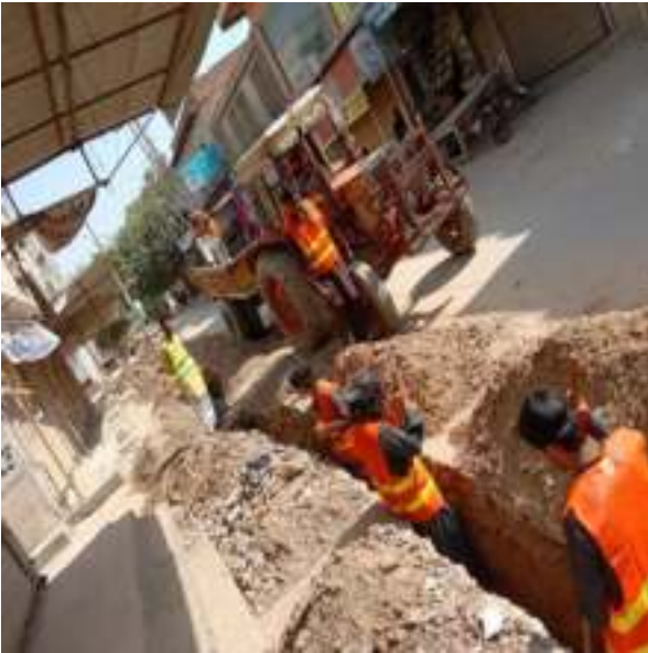
Picture 15: Sand Bedding of Trench AT UC-03
