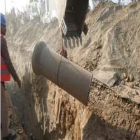
Picture 29: LAYING OF RCC PIPES
