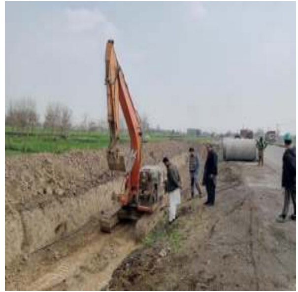
Picture 48: Sewer Bed preparation
