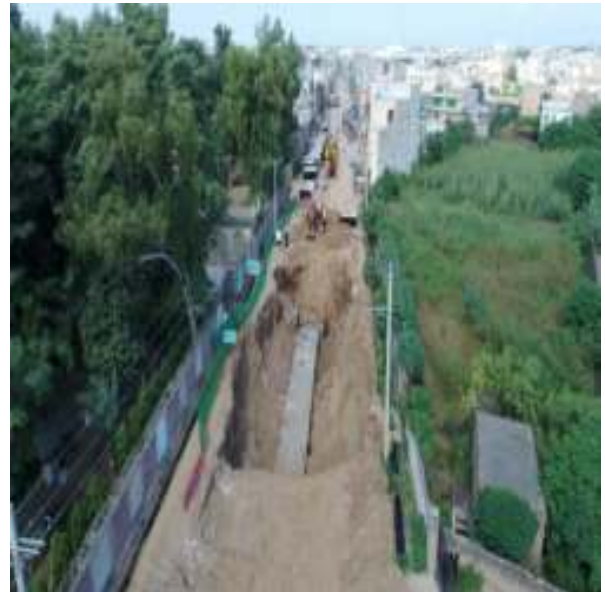
Picture 77: Conduits laying is in progress near Technical College Site 2 Marala Road Sialkot
