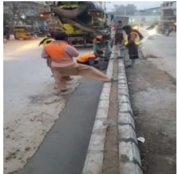
Picture 73: Road Restoration in Process
