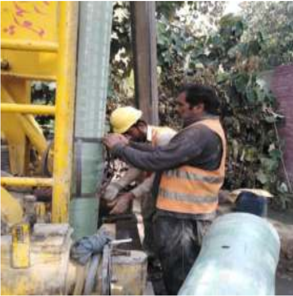
Picture 17: Pipe Lowering of Tube well
