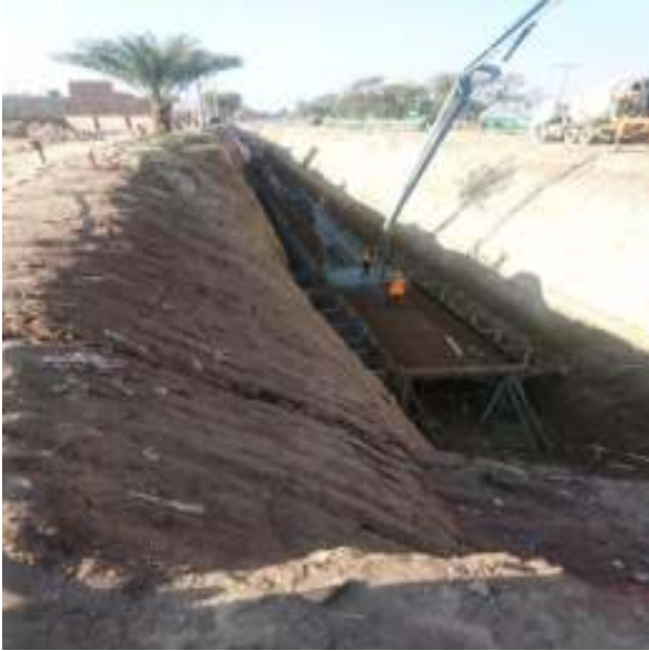
Picture 41: Concrete Roof Slab in Progress, Sahiwal
