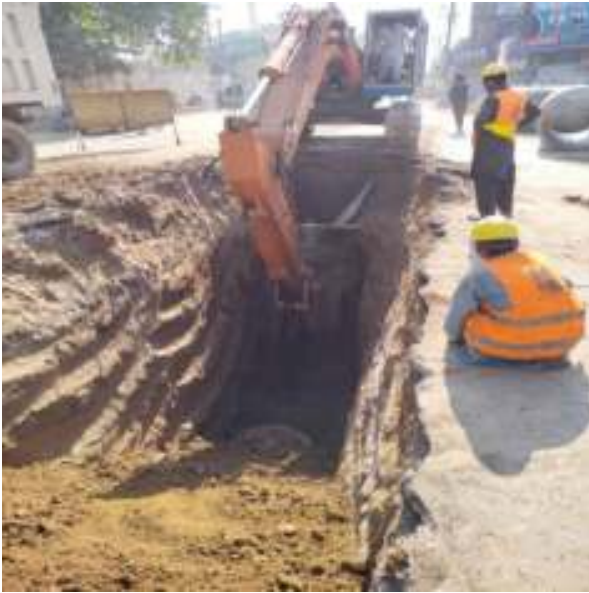
Picture 74: Pipe Laying in Progress
