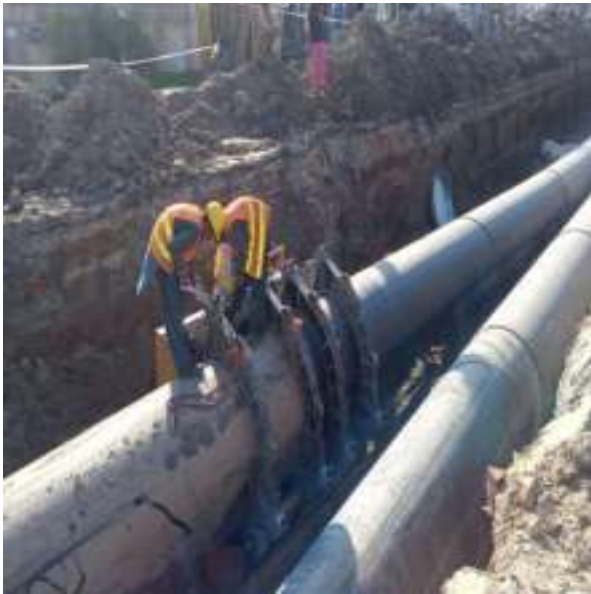
Picture 88: Welding of Forcemain
