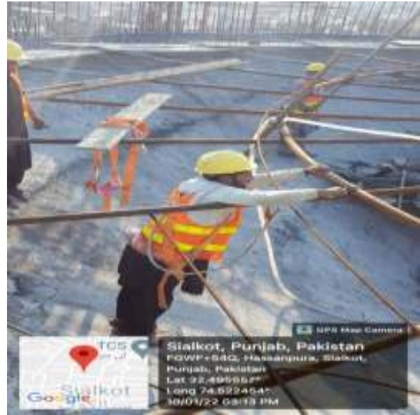
Picture 95: Shuttering Arrangement for OHR
