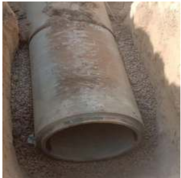
Picture 52: Sewer Laying
