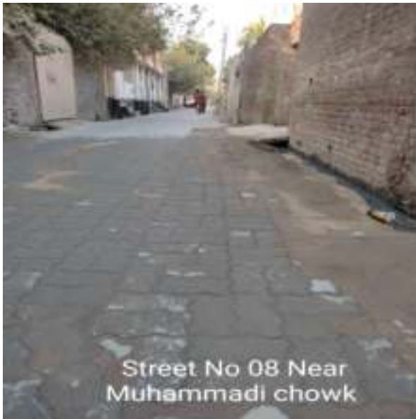
Picture 92: RESTORATION WORKS PICTURES OF LOT-04
