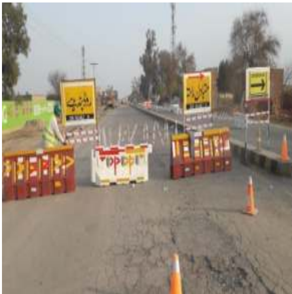
Picture 47: Work in progress and Diversion provided
