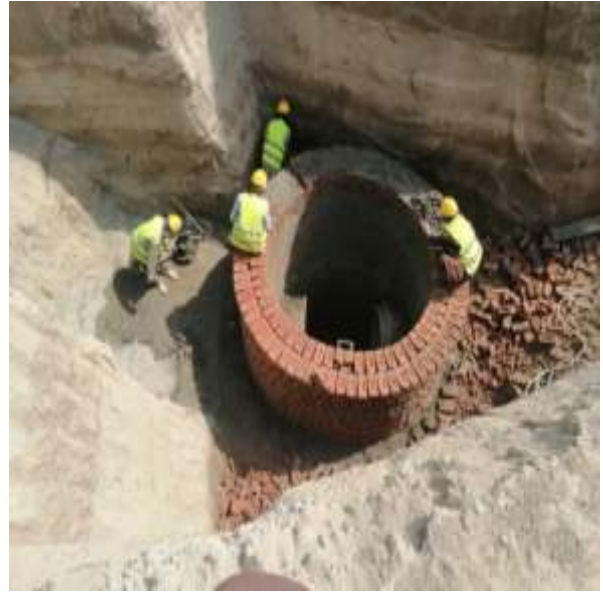
Picture 46: Manhole under Construction
