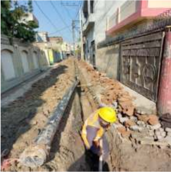
Picture 94: Excavation for Pipe Laying
