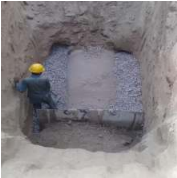
Picture 35: Pipe Bedding with Hunching Lot-02
