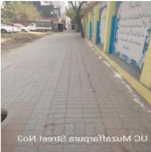
Picture 100: Restoration work at Sialkot
