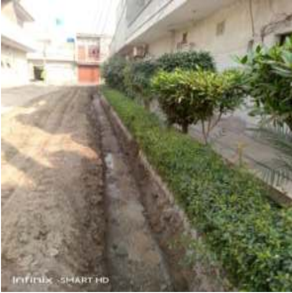
Picture 13: Watering Ramming at Water Supply Lot-01
