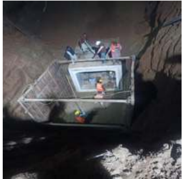
Picture 83: Backfill Restoration
