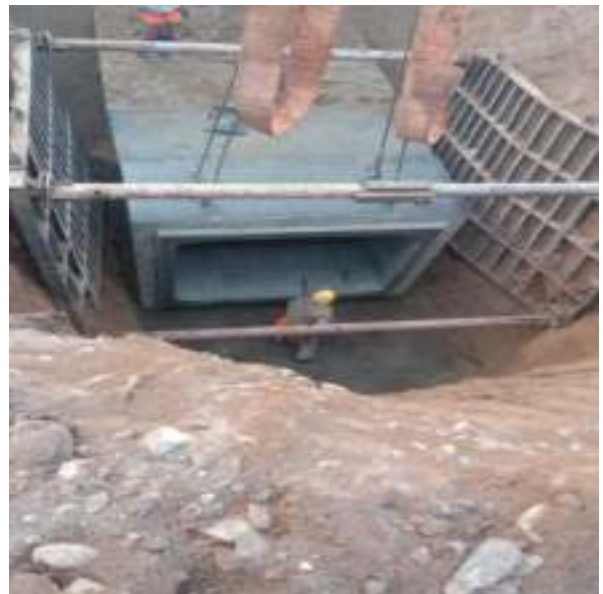
Picture 81: Conduit Laying
