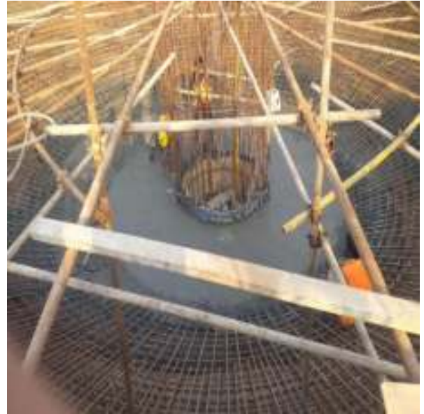
Picture 22: Bowl Concrete Pouring T#7 Ghalla Mandi
