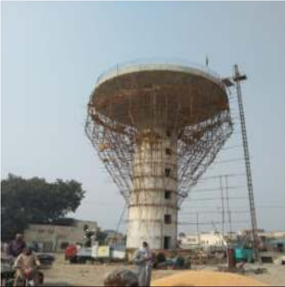
Picture 21: OHR under Construction
