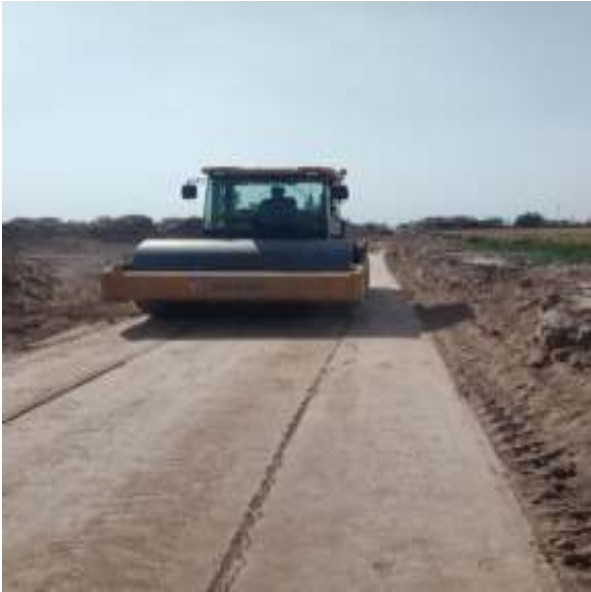
Picture 33: Compaction work is in Progress
