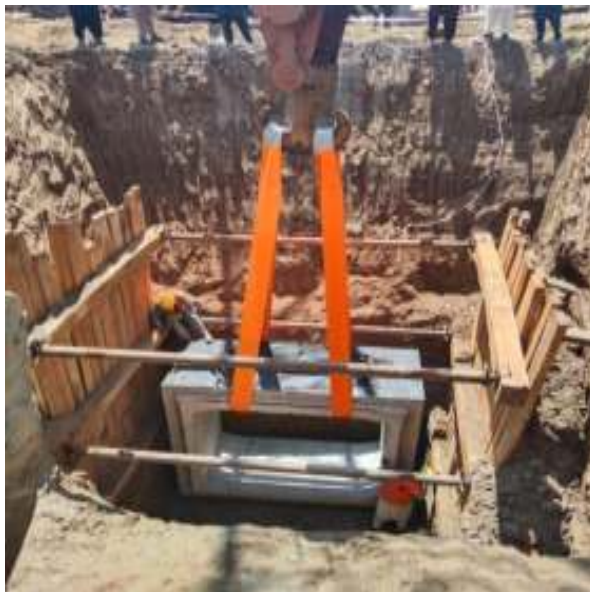
Picture 84: Conduit Placement in Process
