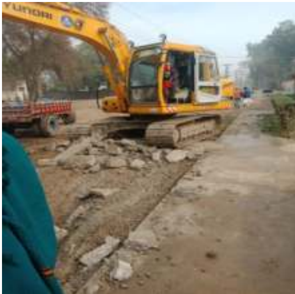
Picture 55: Dismantling of Road-01
