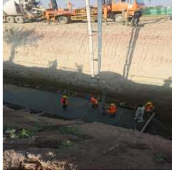
Picture 42: Concrete Roof Slab in Progress, Sahiwal
