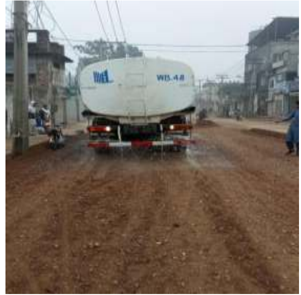
Picture 71: Road Restoration, After Laying of Sewer Line in Process
