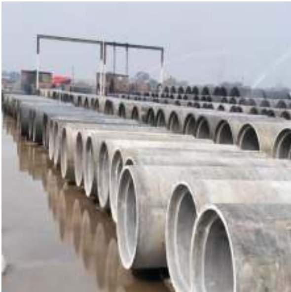
Picture 25: RCC Pipe Curing Yard
