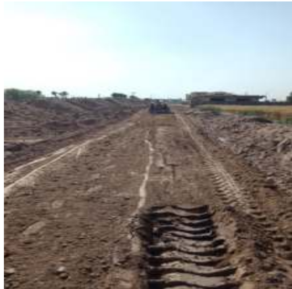
Picture 34: Compaction work is in Progress
