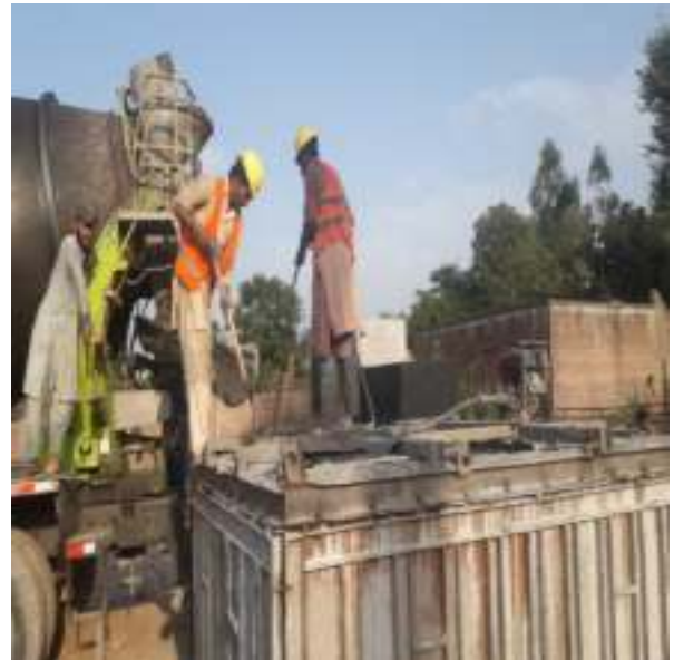
Picture 85: Conduit Manufacturing in Process
