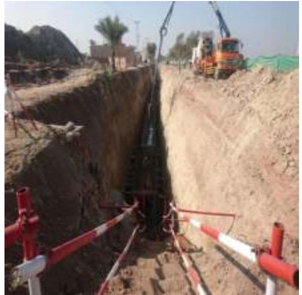
Picture 44: Pouring of Concrete in Progress
